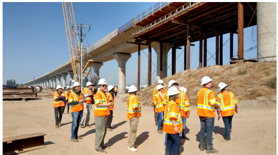
California high speed rail construction site. (Photo: Credit: Mike Christensen)
