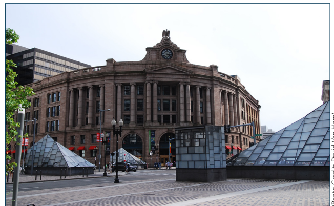
South Station headhouse and subway entrances in Dewey Square.
